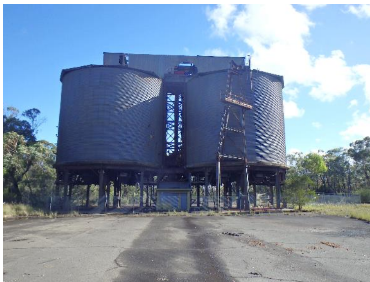
Example of coal loading bins in the Special Area
