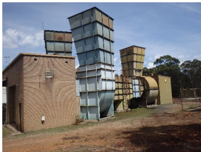
Example of a ventilation shaft site within the Special Area
