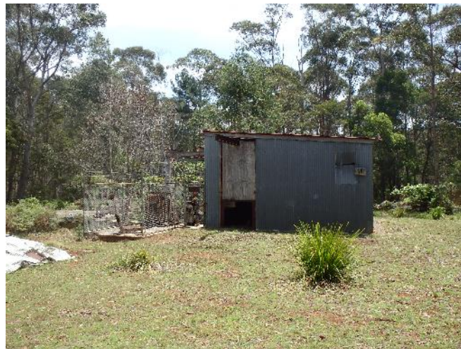
The redundant Nebo No. 3 Shaft
