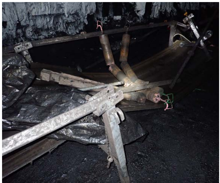
Figure 1 The damaged conveyor structure
