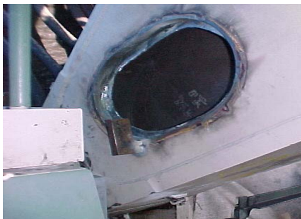
Photo: Box section showing inspection window
