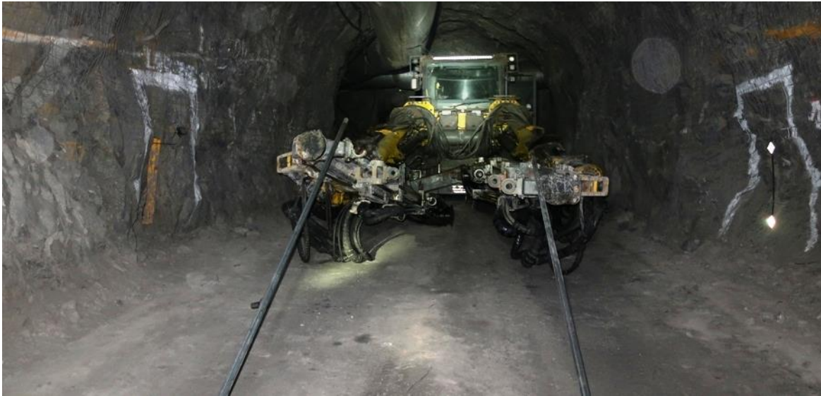
Figure 1. Atlas Copco jumbo parked in the access drive with booms lowered to change drill steels.
