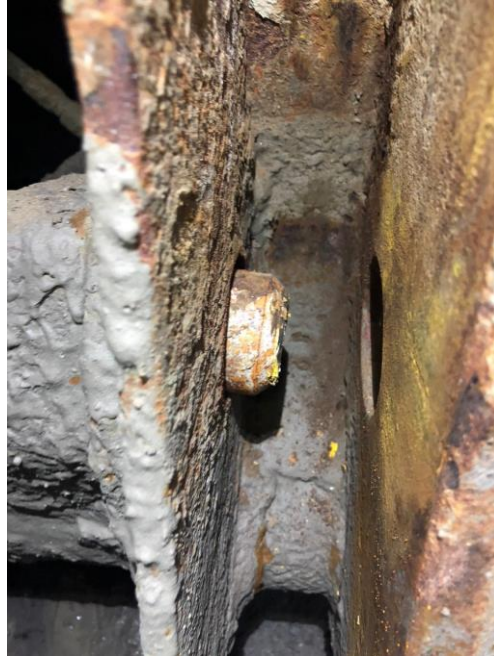
Figure 1. LHS locking pin partially extended
