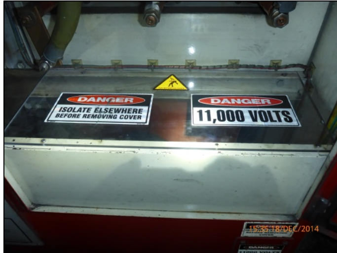
Figure 4: 11000V/110V Control transformer located in bottom of test compartment. Lexan cover removed, as found after the incident.
