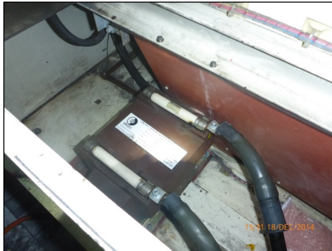
Figure 4: 11000V/110V Control transformer located in bottom of test compartment. Lexan cover removed, as found after the incident.
