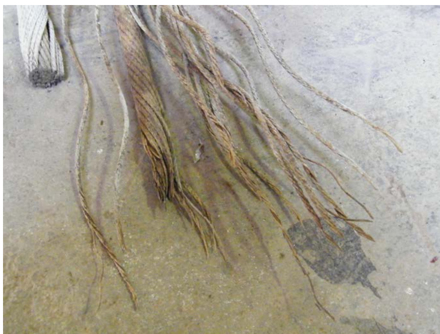
Photo 2 – Close-up of corroded rope.
