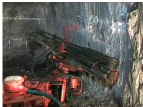
Photograph 4 Reconstruction showing position of the feed beam after the incident
