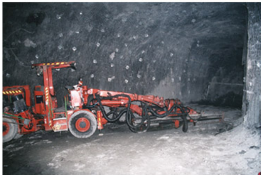
Photograph 1 Side view of the drill jumbo
