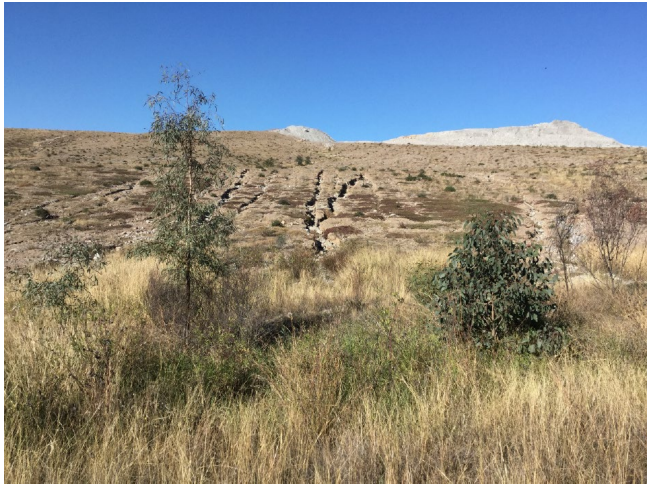
Figure 3 Before - Deep eroded toe drain at the base of the Northern batter of the WEA
