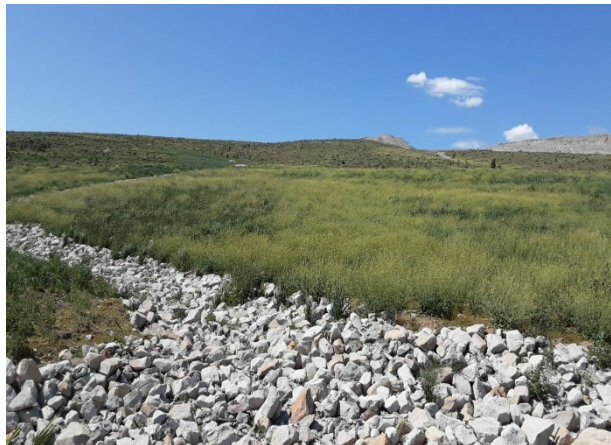
Figure 6 After - Backfilling of gullies and rills. Vegetation establishing on previous identified bare patches
