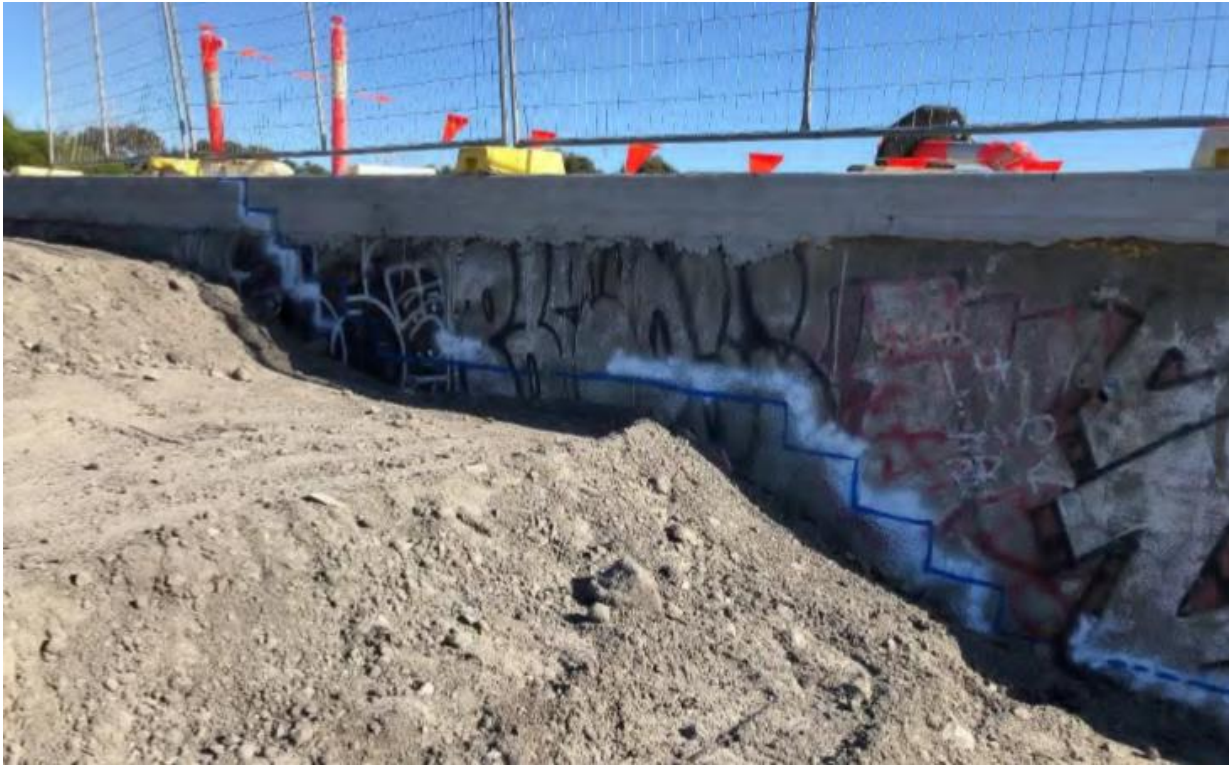
Figure 18: Completed capping of the second pier of the coal bin site (February 2021)
