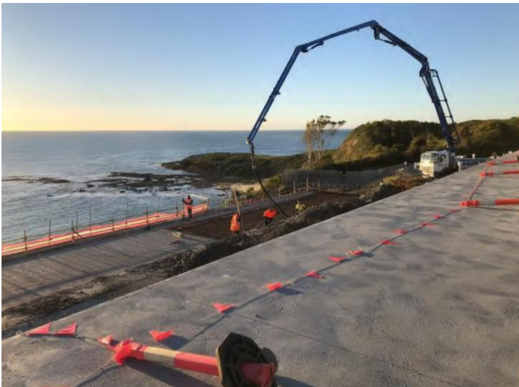
Figure 16: Pouring of final capping slab of third pier of the coal bin site (July 2020)
