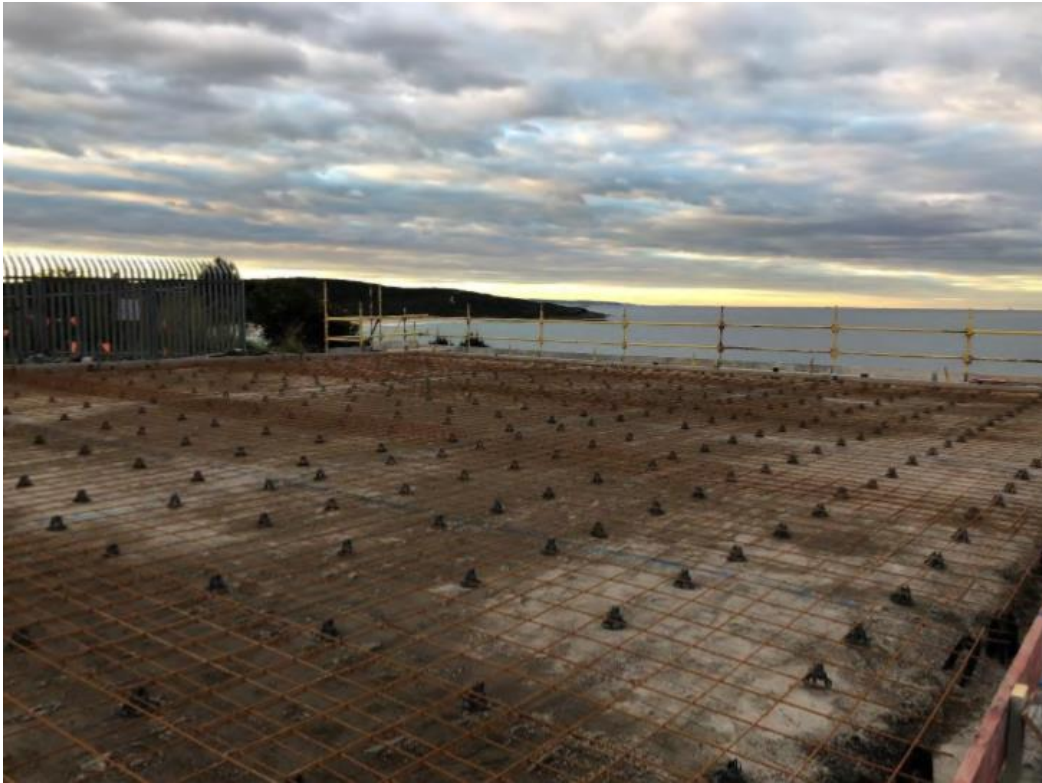
Figure 16: Pouring of final capping slab of third pier of the coal bin site (July 2020)
