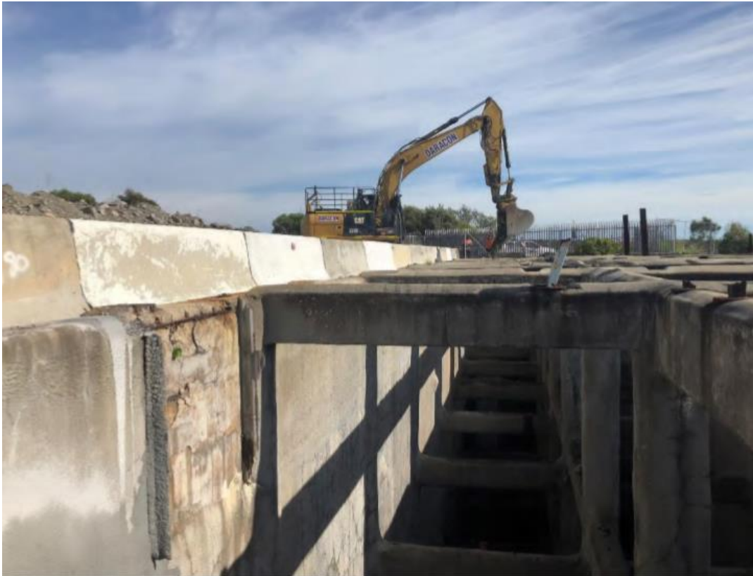
Figure 13: Coal bin filling works including placement of crushed hardstand material ('rubble') (April 2020)
