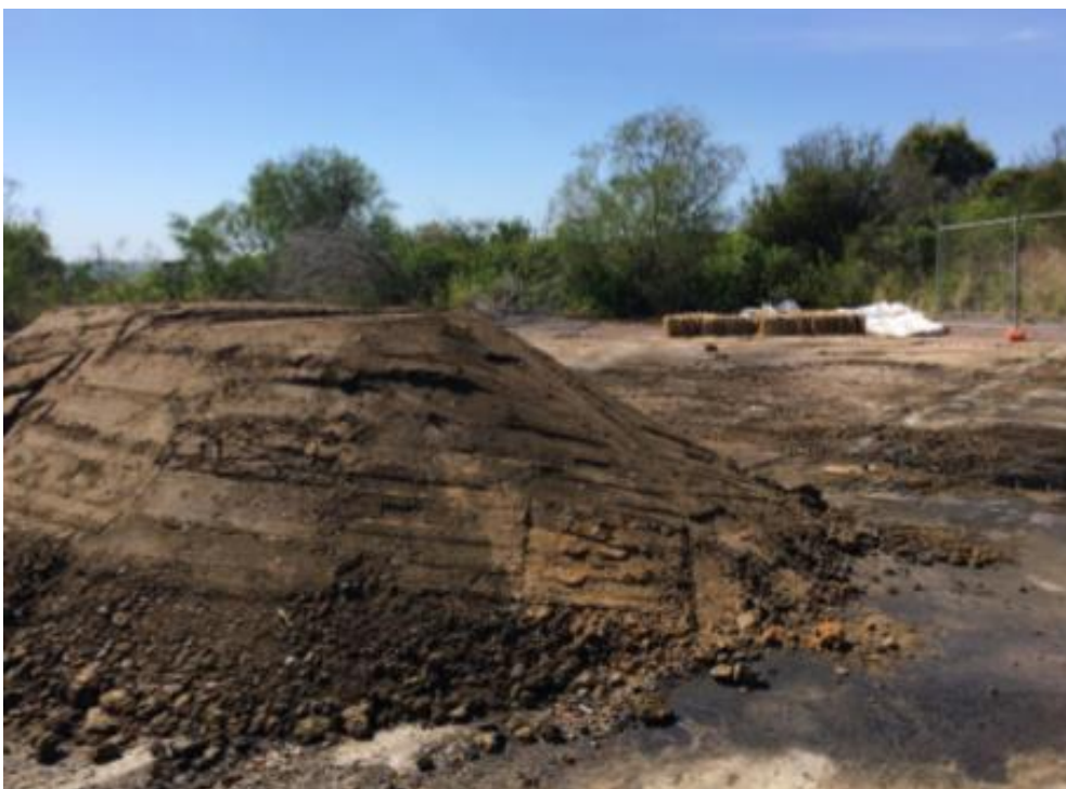
Figure 10: Stockpiling of hydrocarbon contaminated material for bioremediation (2016)
