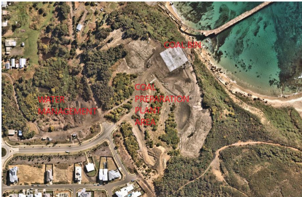
Figure 8: Domains 1A, 2A and 4A in September 2020 finalisation of coal bin filling works to produce a terraced viewing platform, finalisation of associated drainage control measures and installation of balustrade and associated fencing. Filling works achieved up to 35MPa compressive strength that has been independently verified. Weed control efforts also performed.
