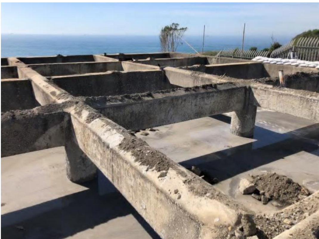
Figure 14: Pouring of grout / cement slurry within coal bin site (April 2020)
