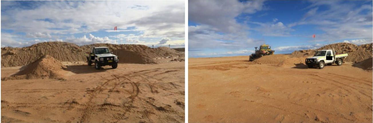
Figure 11: BSL Dozer and light vehicle parked up at light vehicle/light tower bund
