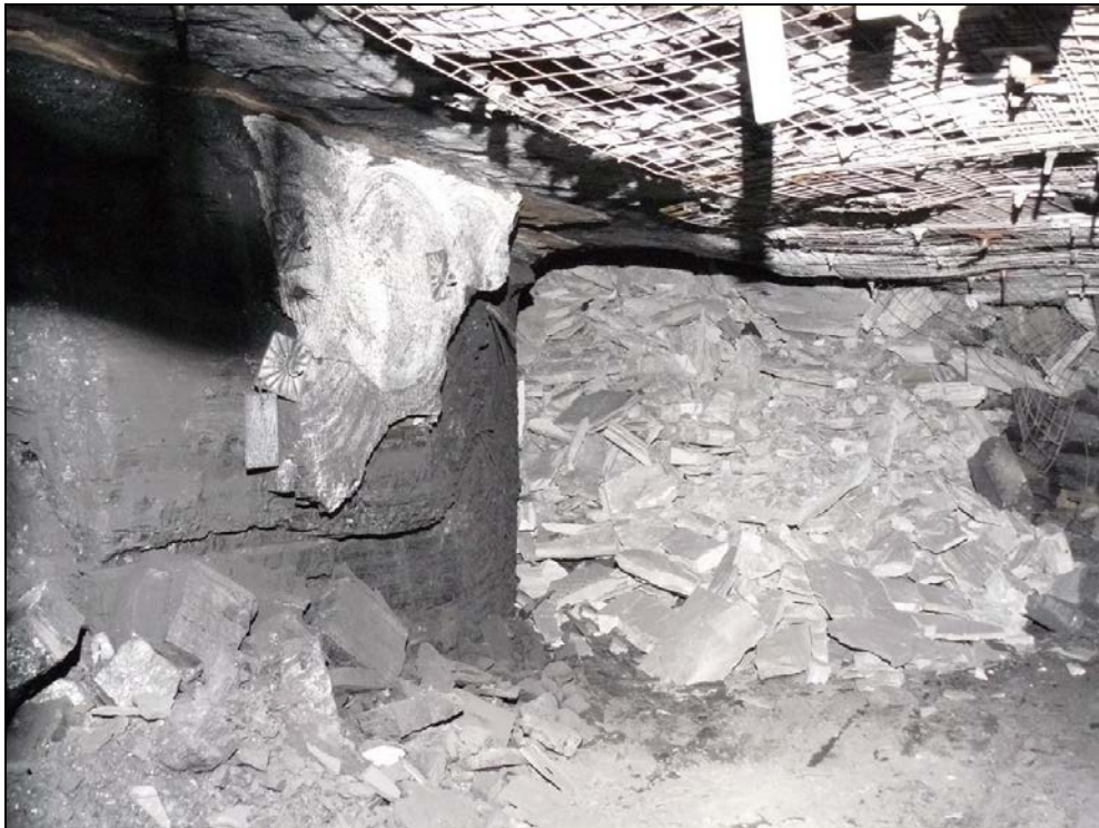
Photograph 18 View looking inbye of 6 cut-through inbye the breaker line support position showing rib support in left hand side rib and goaf edge at 6 cut-through in B Heading.
