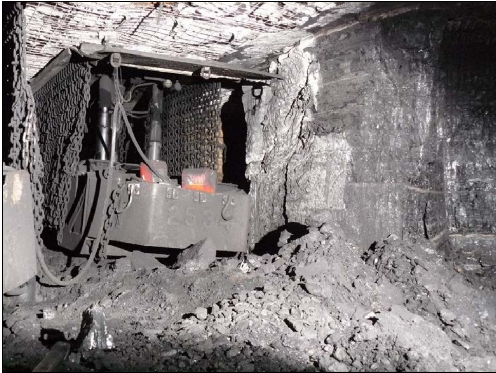
Photograph 16 Looking inbye of the right hand side breaker line support in relation to the start of the right hand side rib pocket.
