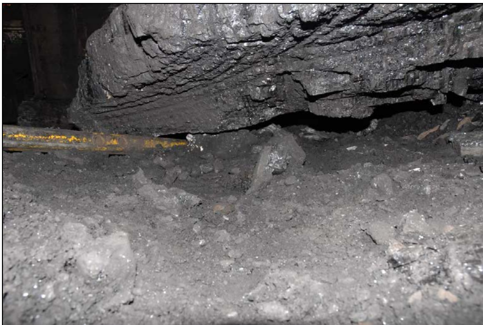
Photograph 12 Underside view of slab showing the position of steel belt clamp.
