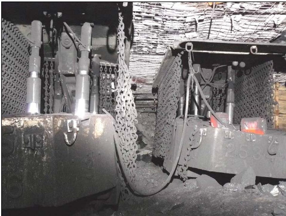
Photograph 17 Looking inbye of the position of the two breaker line supports towards the goaf edge.
