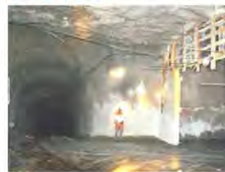
Photo depicting height of water during inrush
