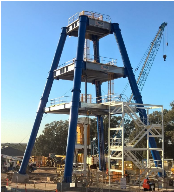
Figure 12 Headframe for a typical stage winder
