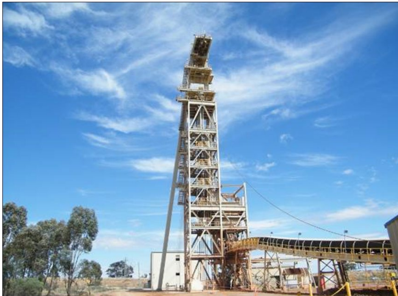
Figure 8 Ground-mounted friction winder
