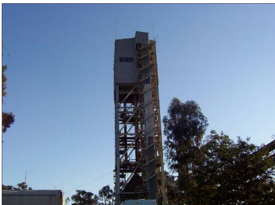
Figure 7 Tower-mounted friction winder house
