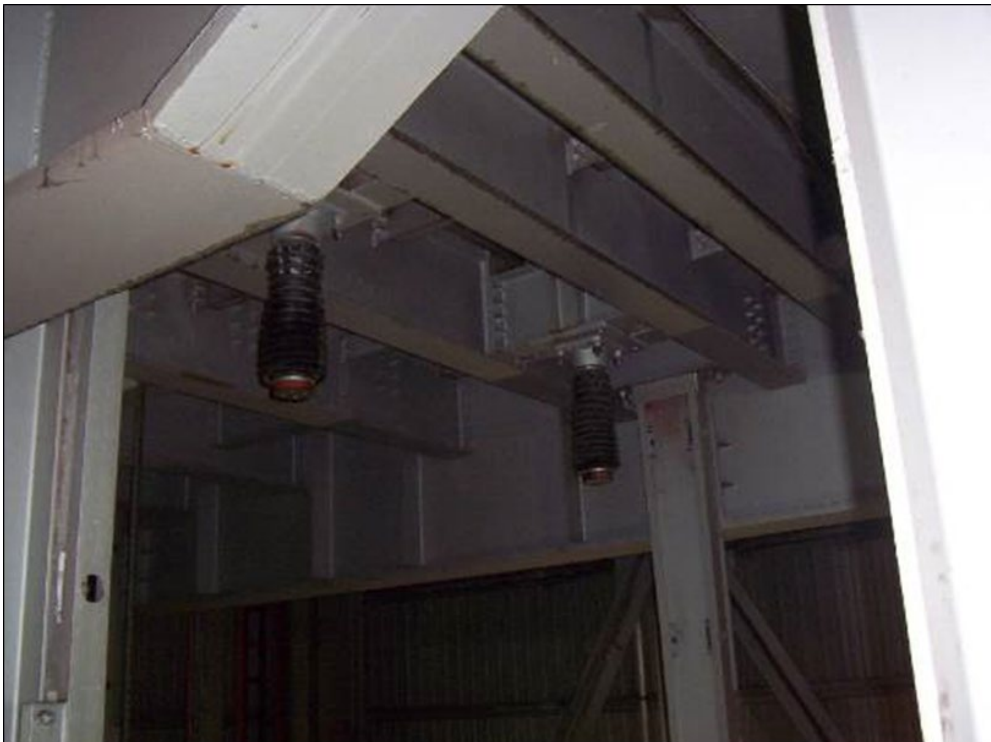
Figure 25 Arresting device in vertical shaft headframe
