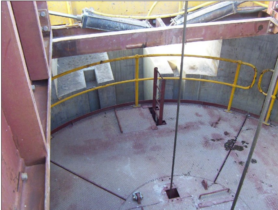
Figure 17 Top deck of stage in shaft below surface collar
