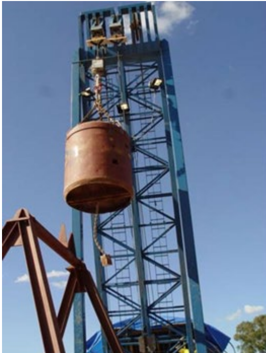
Figure 15 Kibble winder and kibble suspension
