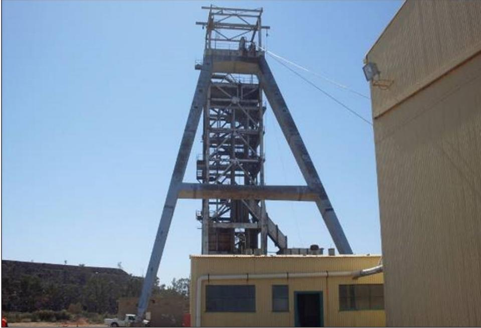
Figure 14 Headsheave installation - drift winder
