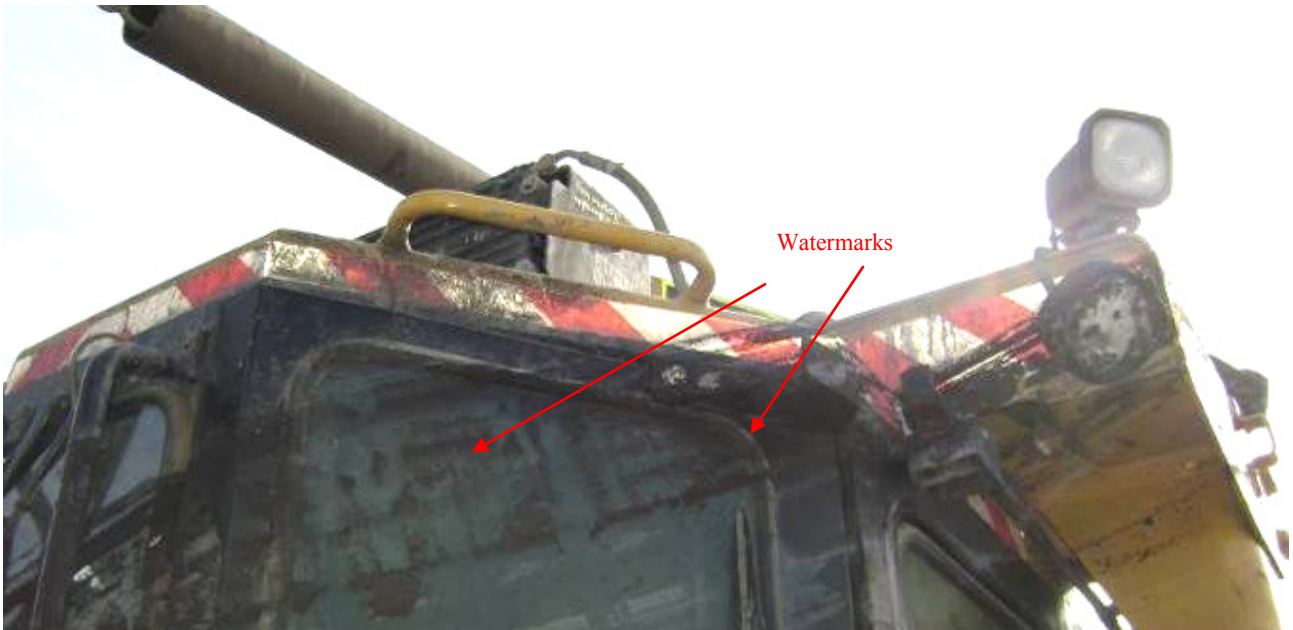
Photograph 7: Water mark at the top of the external part of the cabin of the dozer 4 .
