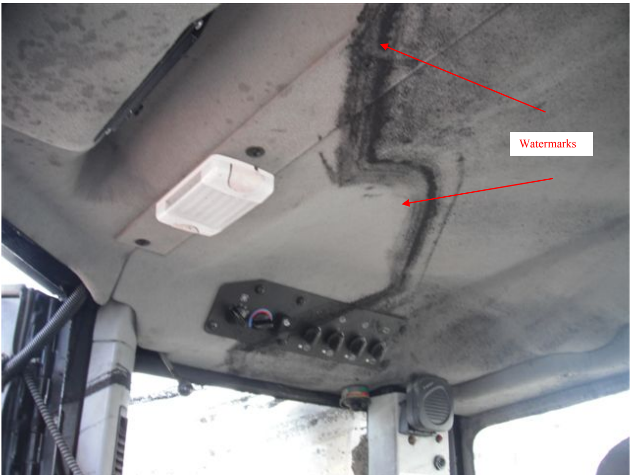
Photograph 8: Inside the cabin of CAT D11T dozer showing water mark on the ceiling 5 .
