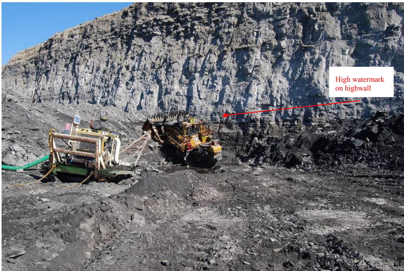
Photograph 9: CAT D11T dozer in the sump after water was pumped out.
