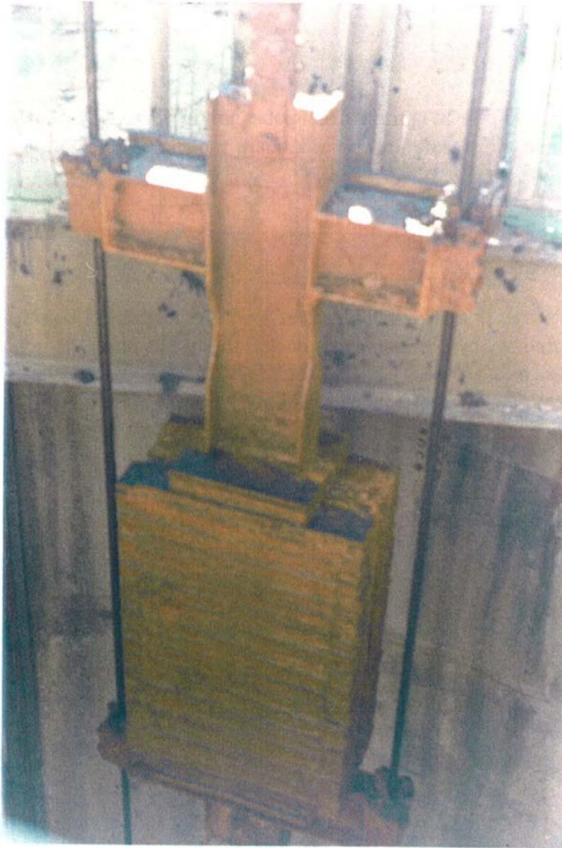
Vertical shaft winder counterweight
