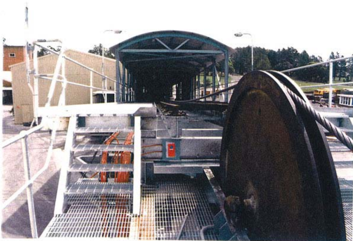
Headsheave Installation - Drift Winder
