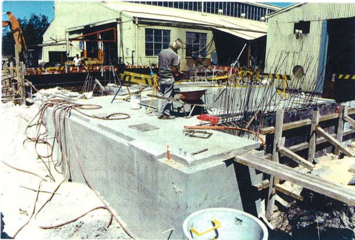
Winder foundations showing pit and footings.
