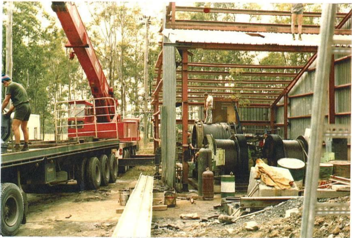
Shaft Sinking Winder under construction
