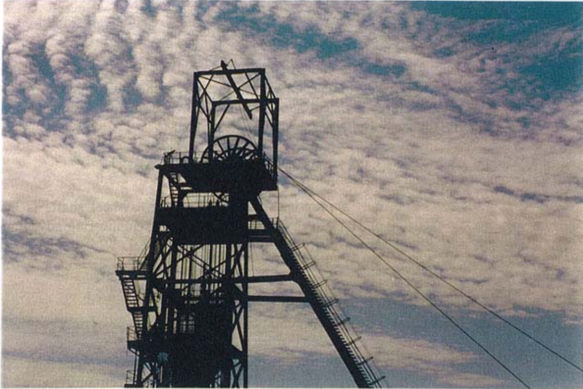
Headsheave Installation - Shaft winder
