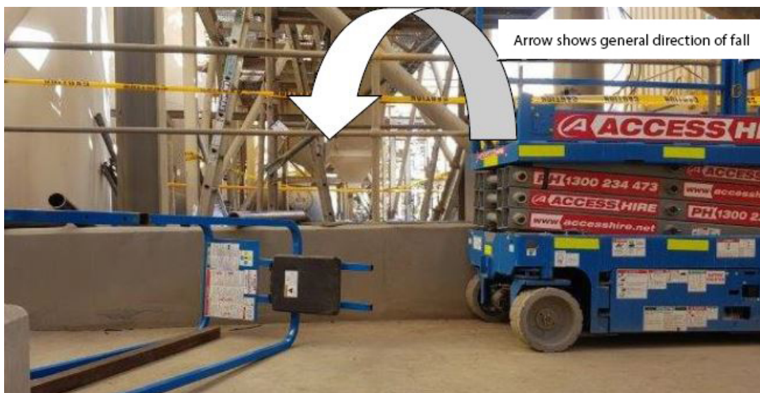
Figure 1 Direction of fall and guardrail on ground
