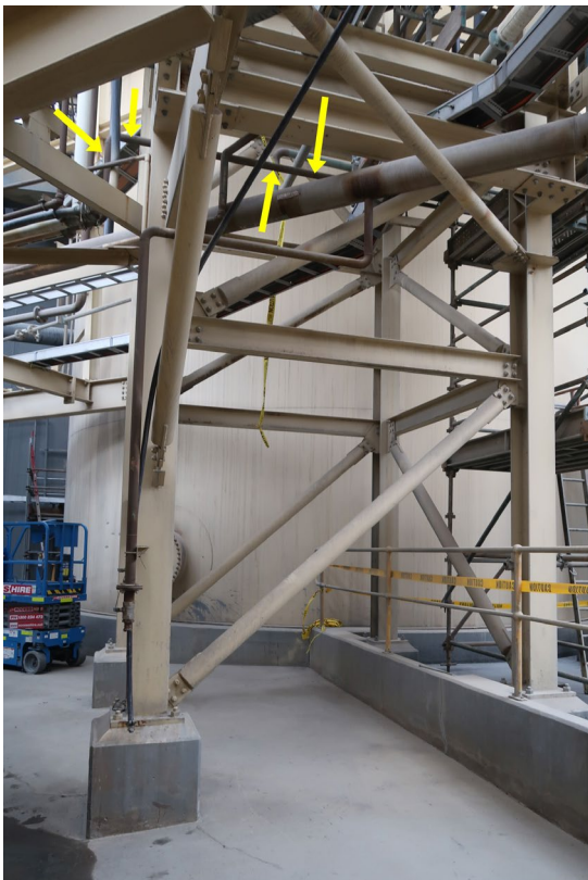
Figure 9 Required location of pipe within structure
