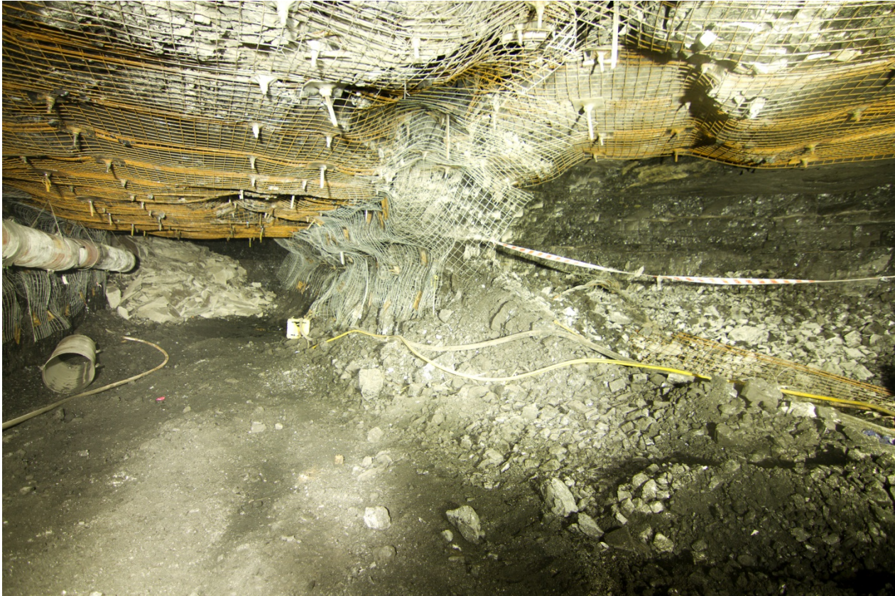
Figure 9 The 'stub' heading showing where CM 35 withdrew from before returning to B Heading.
