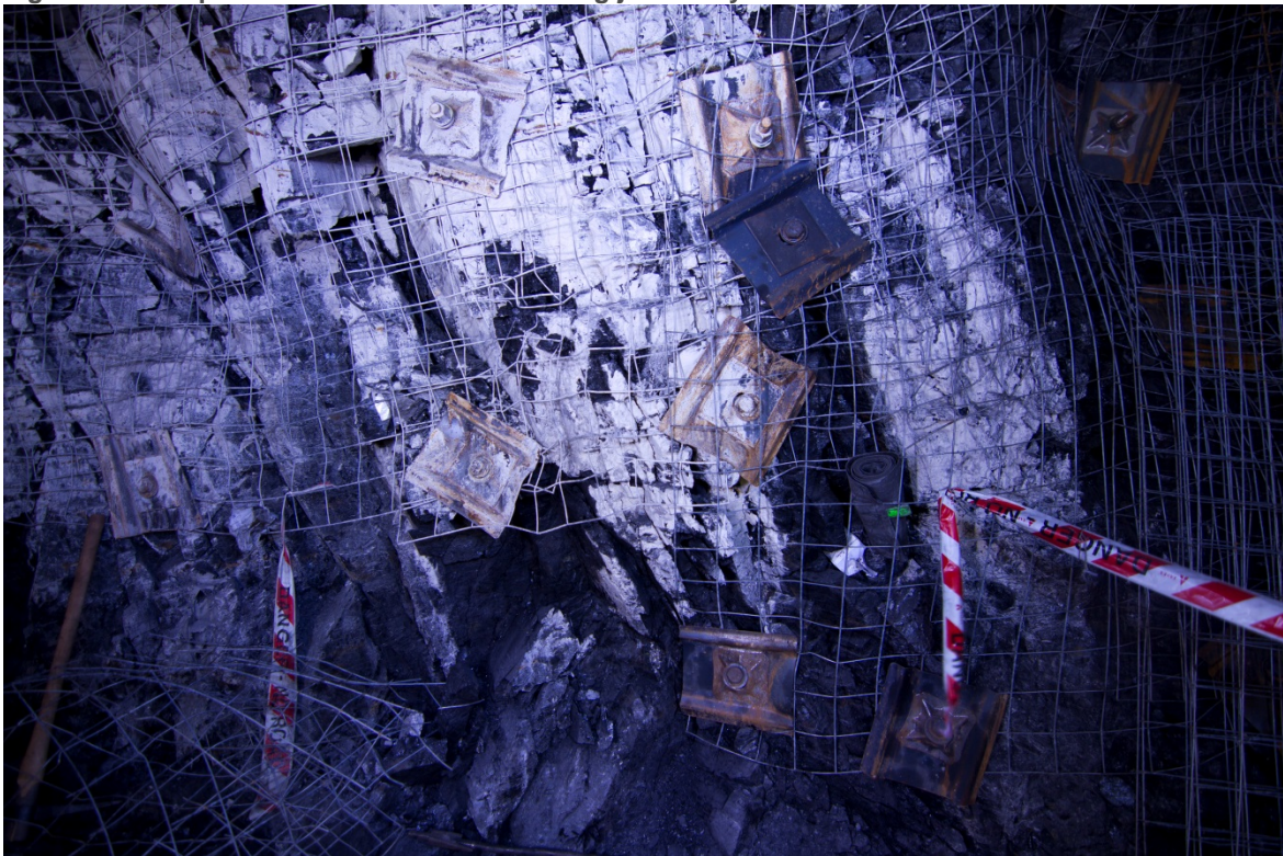
Figure 25 Example of rib bolts LHS of B Heading just outbye of the incident.
