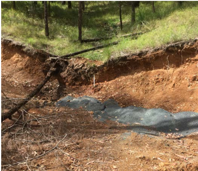
Figure 3 Poor drill cutting management
