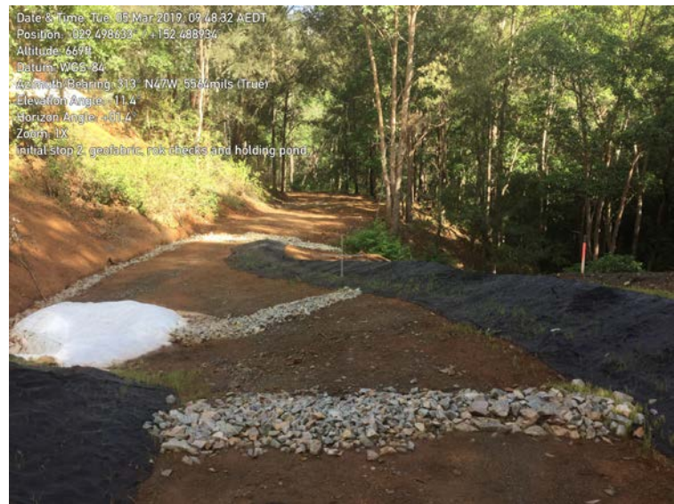
Figures 6 and 7 Effective use of sediment and erosion controls in the form of rock checks and geofabric
