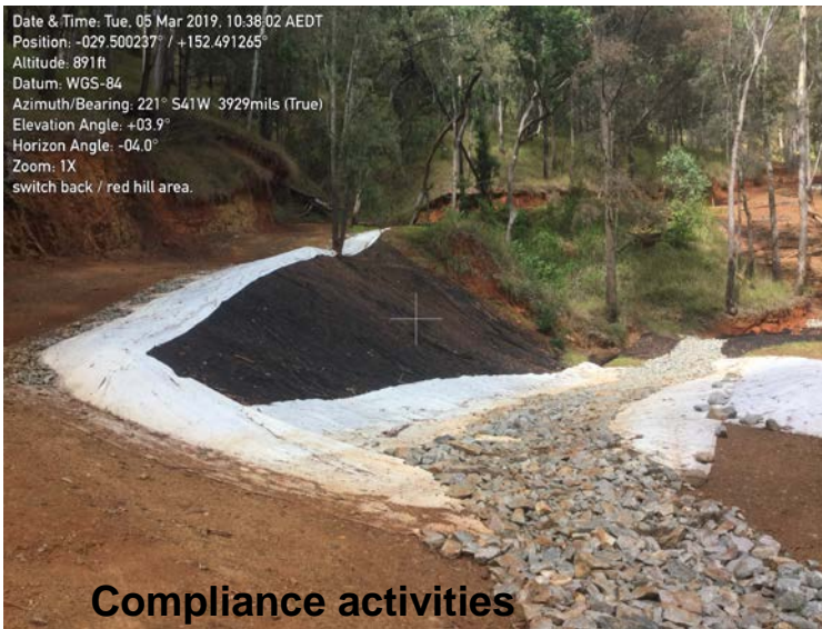
Figures 6 and 7 Effective use of sediment and erosion controls in the form of rock checks and geofabric
