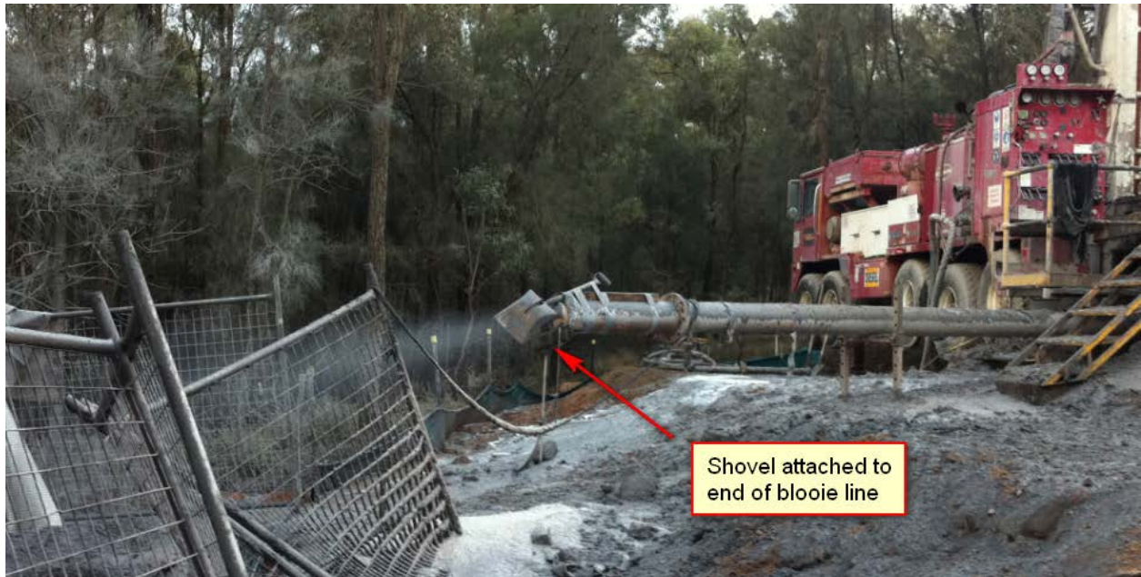
Blooie line at borehole 3 passing under the driller's platform
