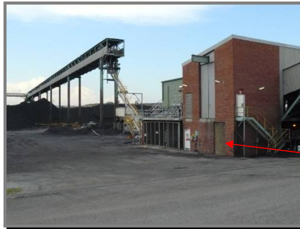
Photo shows UTL Building, with UTL switch room below
