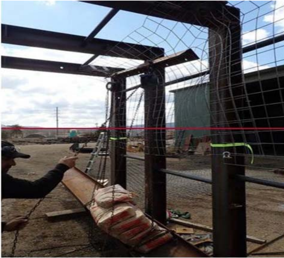
Testing Lightweight Rib Mesh
