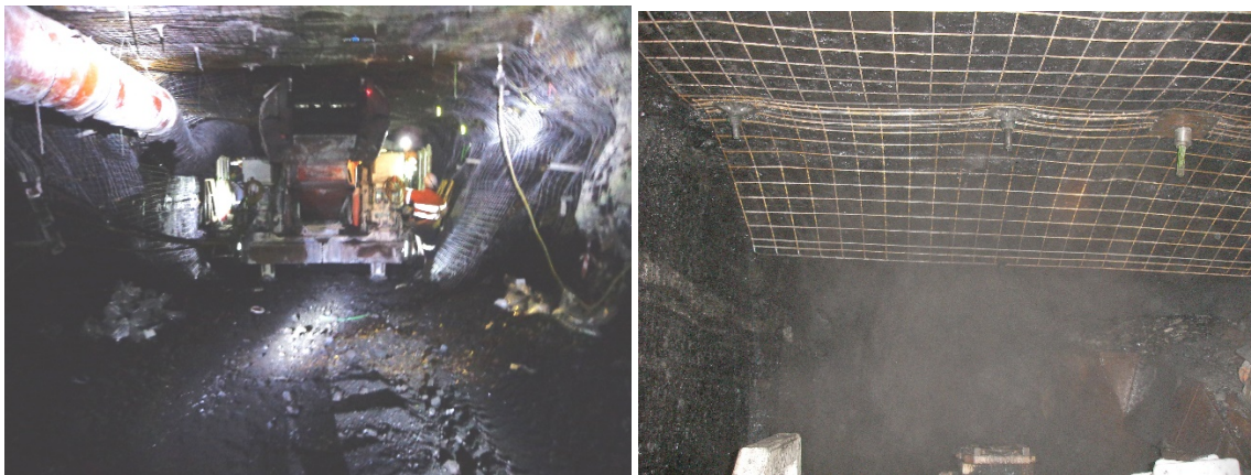
Fig 8: Photos of underground roof bolting.
