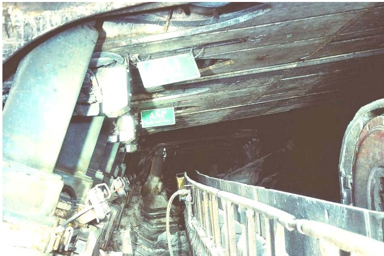
Figure 18: Longwall as it looked on re-entry
