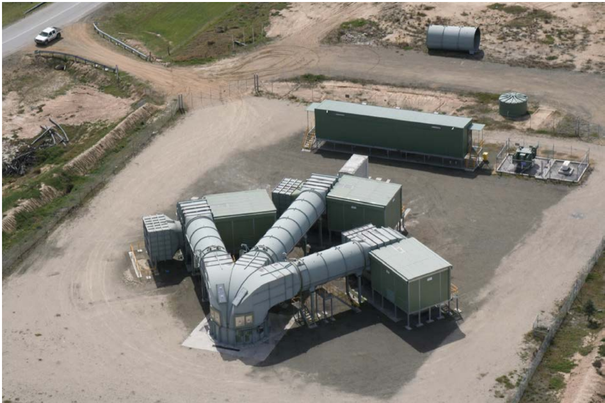
Figure 5: No 1 shaft fan installation 9
