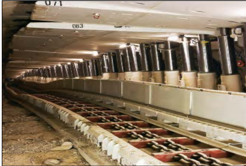
Figure 1: Typical longwall face showing chocks and AFC
