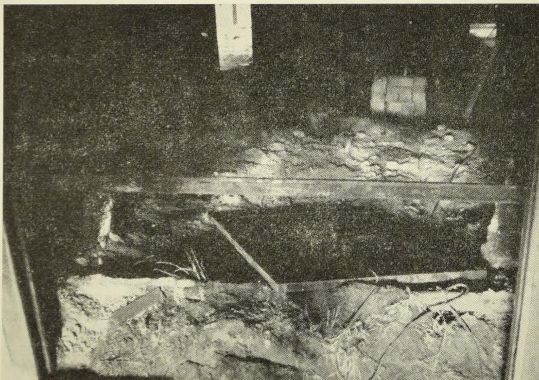
Seal over upcast shaft. (24th December, 1963.)
