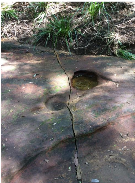
Figure 10 Cracking in creek bed at edge of LW31 near logger R9
