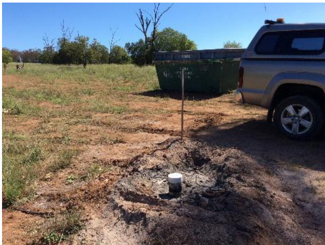
Figure 5 Metal skip bins for drill cuttings ready to be relocated to next chip hole
