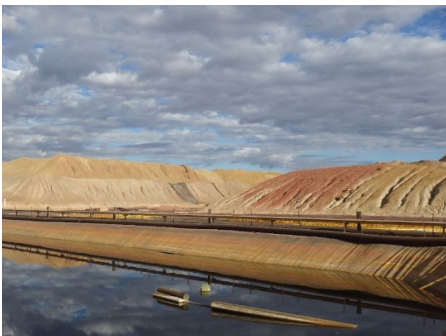
Figure 5 Heap leach pads and pregnant liquor pond at Murrawombie Mine
