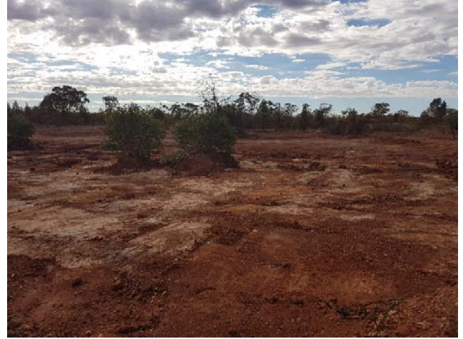
Figure 9 Remediation of the water pipeline spill area
