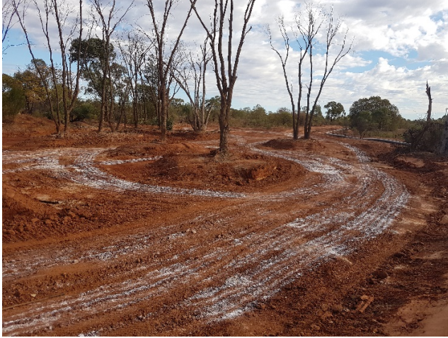
Figure 8 Remediation of the water pipeline spill area
