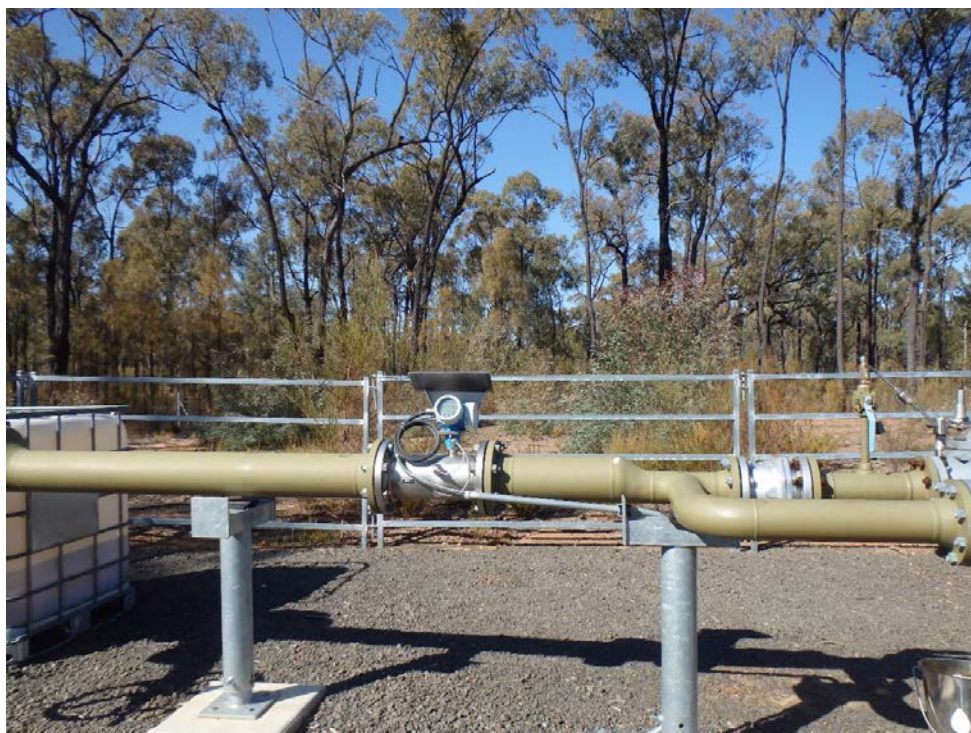
Photo 2: Ultrasonic gas flow meter installed on the flare line at Dewhurst 28.
