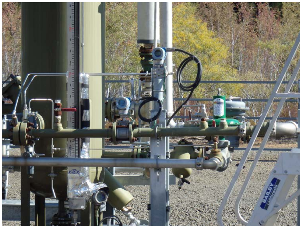
Photo 2: Ultrasonic gas flow meter installed on the flare line at Dewhurst 28.
