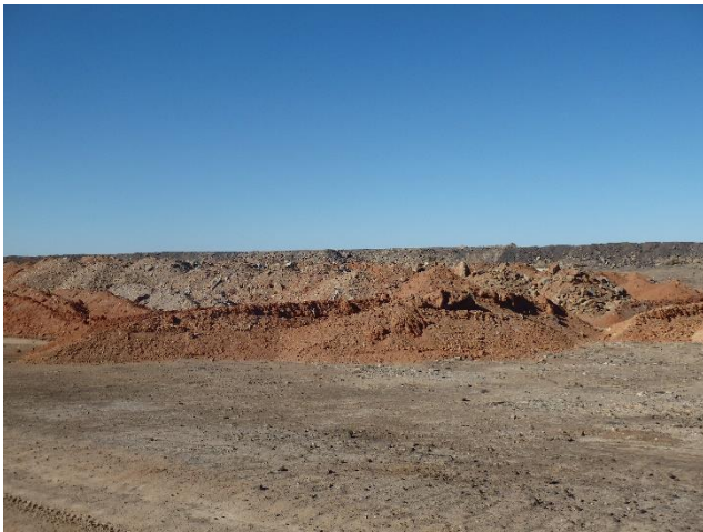
Figure 5 Topsoil stockpiled on the top of a waste emplacement at North Mine
