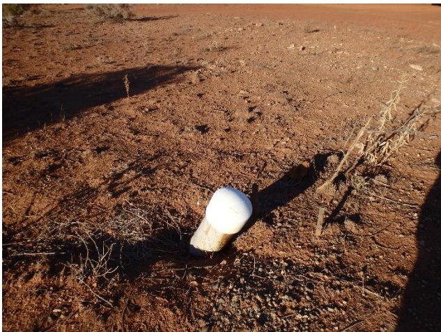
Figure 19 Hole drilled in 2008, casing still extending above ground level
