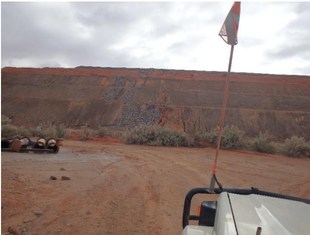
Figure 4 Erosion on the embankments of former TSF Site A-B
