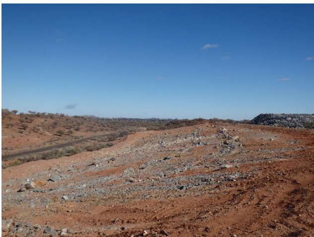
Figure 6 Batters of the Potosi WRE reshaped and ripped
