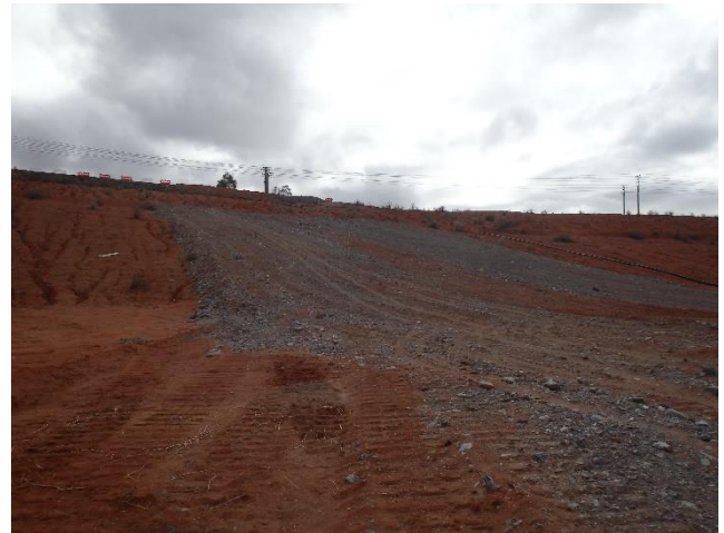
Figure 3 Waste rock being used to rock armour the TSF embankment
