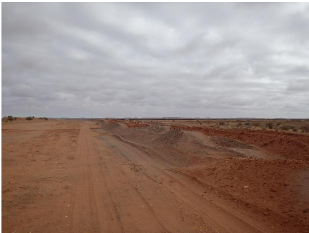
Figure 1 Windrowed topsoil stockpiles on cell 1 Site D TSF
