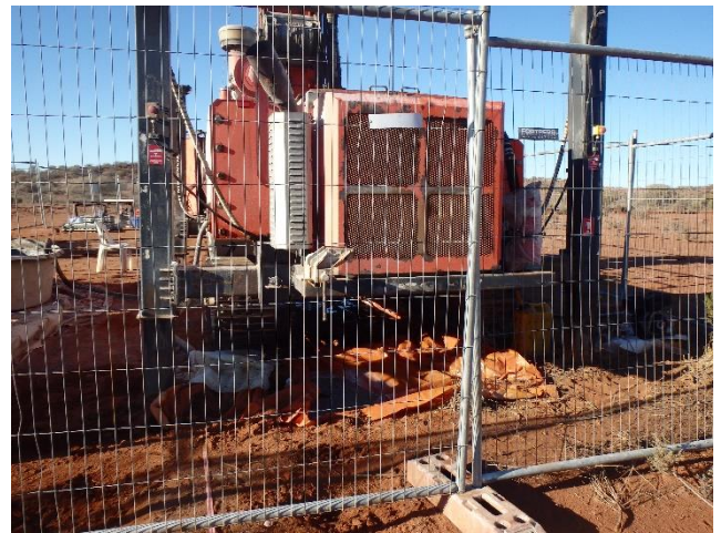
Figure 18 Use of spill control matting under the drill rig
