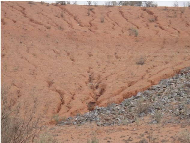
Figure 4 Erosion on the embankments of former TSF Site A-B
