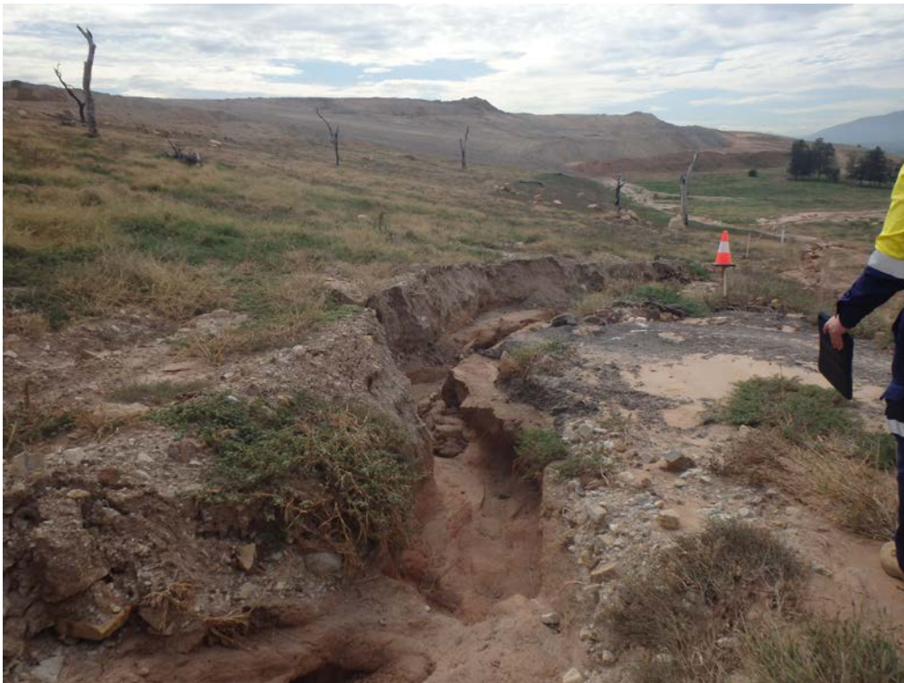
Figure 3 Significant erosion in the overburden emplacement rehabilitation area
