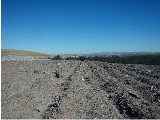
Figure 6 Loosely placed topsoil and mulch in stockpile 14
