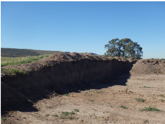
Figure 8 Topsoil recovery from stockpile 19
