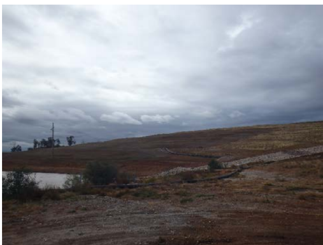
Figure 2 An area of Riverview North where topsoil was direct placed
