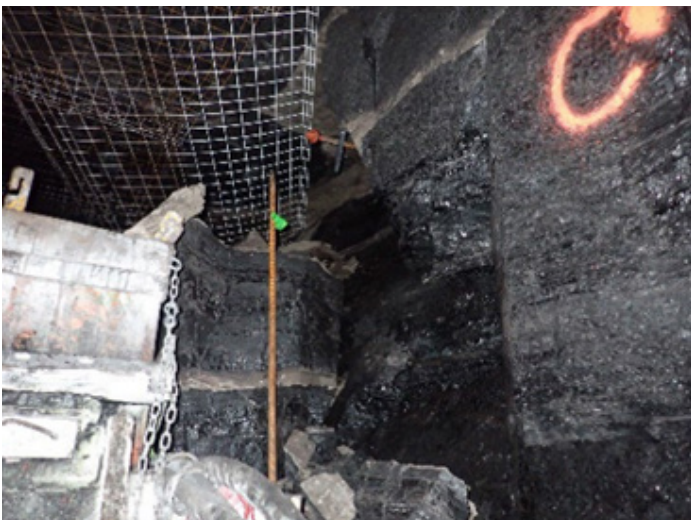
Picture 1. Rib fall in panel
