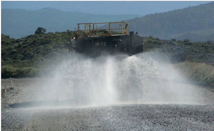
Figure 4: Dust suppression using a mobile tanker.
