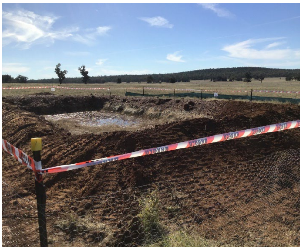
Figure 1 Sump where bund wall was removed
