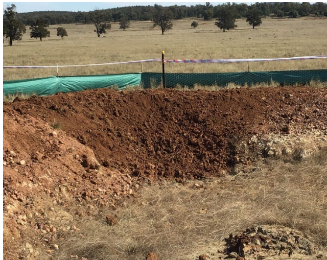
Figure 2 Remedial action taken at sump
