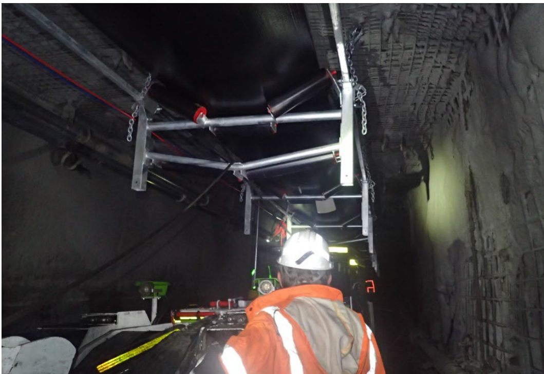
Figure 3 – Re-enactment of rope pulling through conveyor structure
