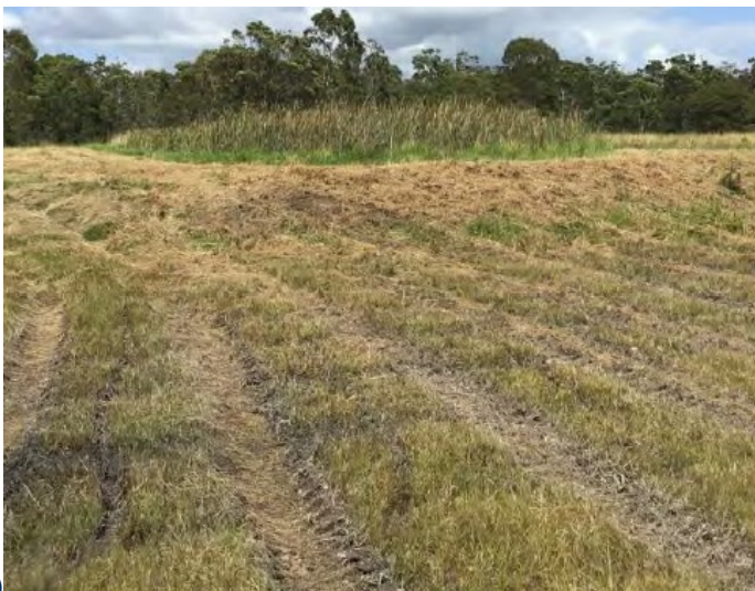
Figure 12: Vegetated tailings dam cap and 'turkeys nest' central dam (2022)
