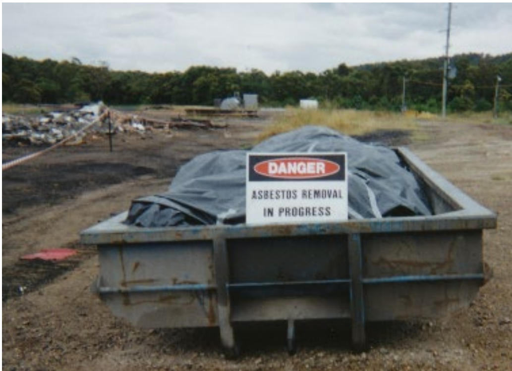
Figure 3: Removing asbestos contaminated demolition materials (circa 1999)
