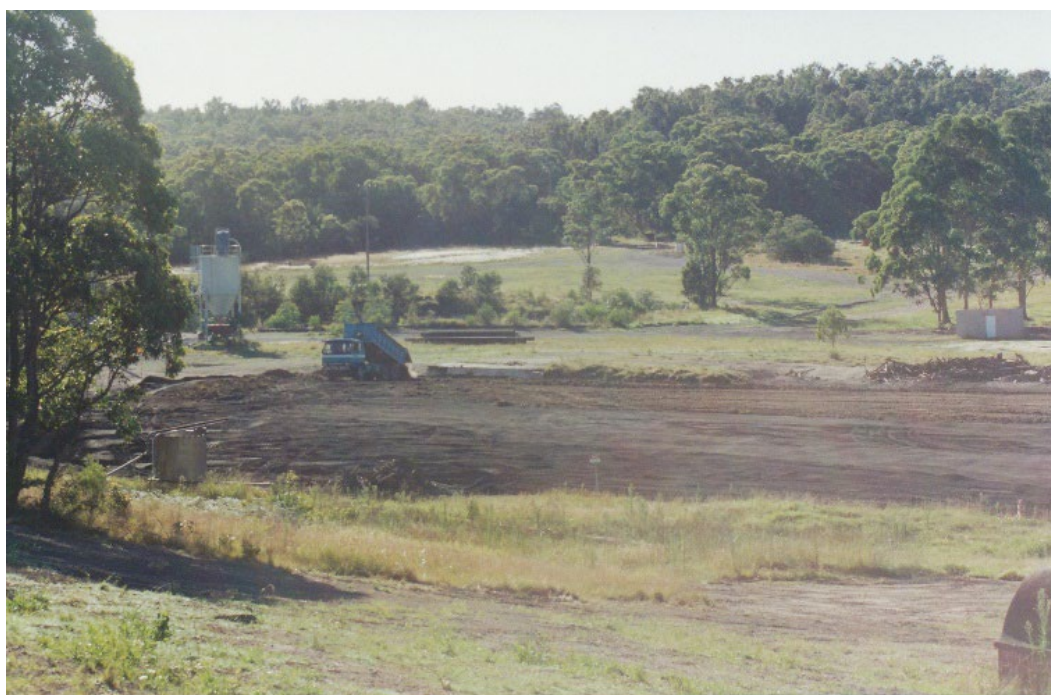
Figure 9: Topsoil spreading over coarse rejects for final planting (circa 2000)
