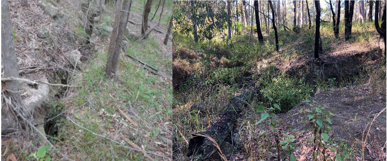
Figure 11: Remediation of subsidence cracks following grouting (circa October 2022)
