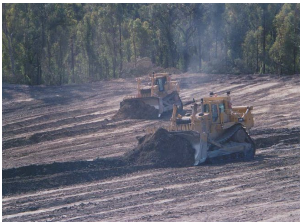
Figure 7: Reshaping of main open cut area (2004)
