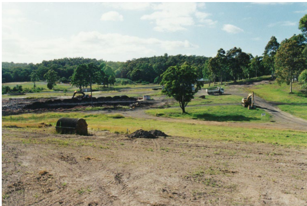
Figure 9: Topsoil spreading over coarse rejects for final planting (circa 2000)
