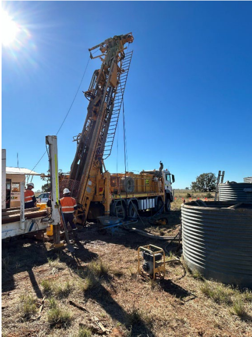
Figure 1 Drill rig set up at DCKDH018
