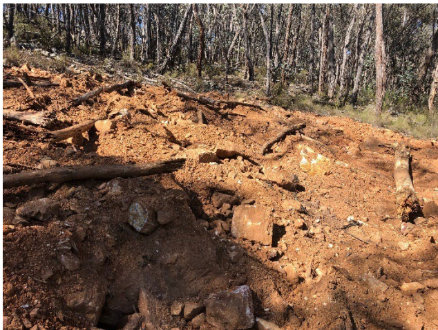
Figure 3 Drill pad Q constructed in 2022 but not drilled, rehabilitation earthworks completed in September 2023
