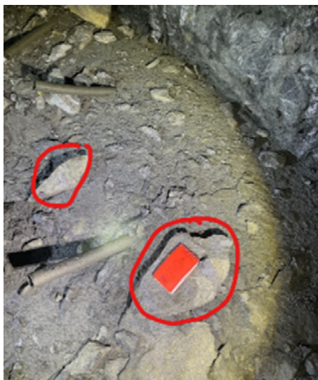
Picture 3. Rock that fell during the incident.
