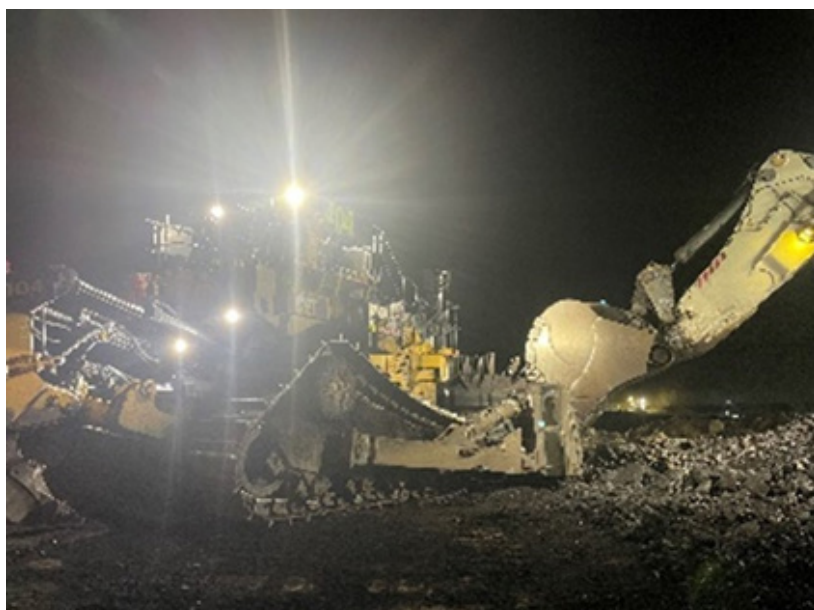
Picture 8. Dozer following the incident.
