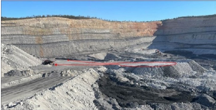
Picture 10. Scene of the incident.
