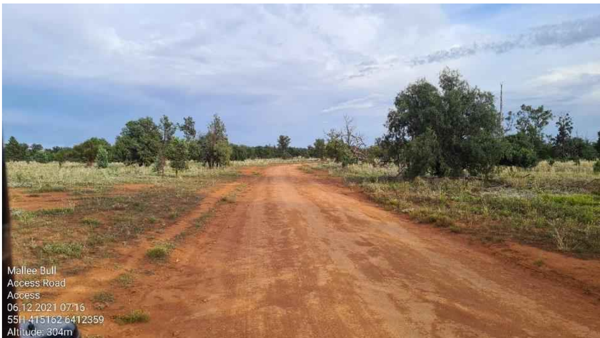
Photo 3: Existing southern site access road
