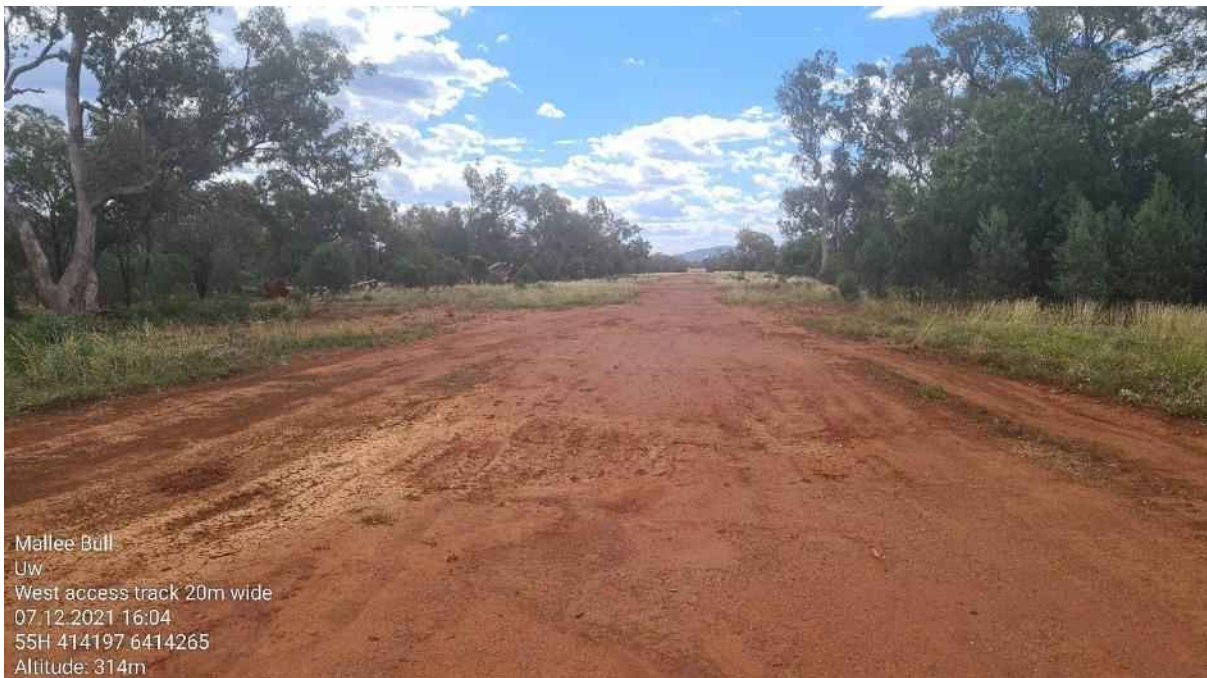
Photo 1: Existing western site access road
