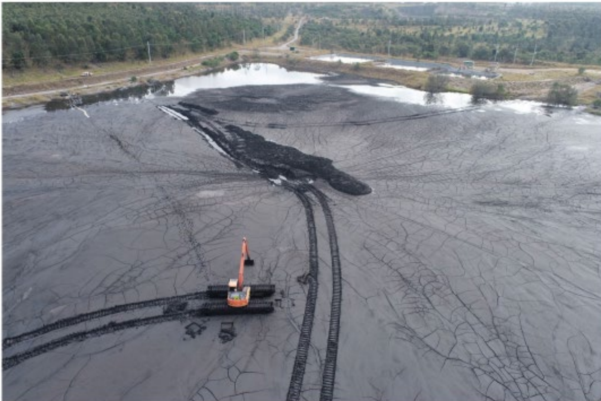
Figure 1: Amphibious excavator stranded on the active tailings dam.
