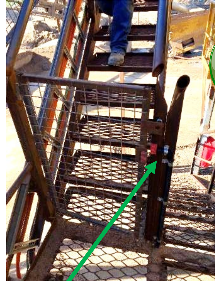
Interlock on gate (plant must need to be restarted if opened) What if others close the gate and restart? How is personal isolation applied?
