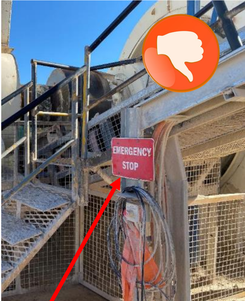
Emergency Stop clearly signposted
