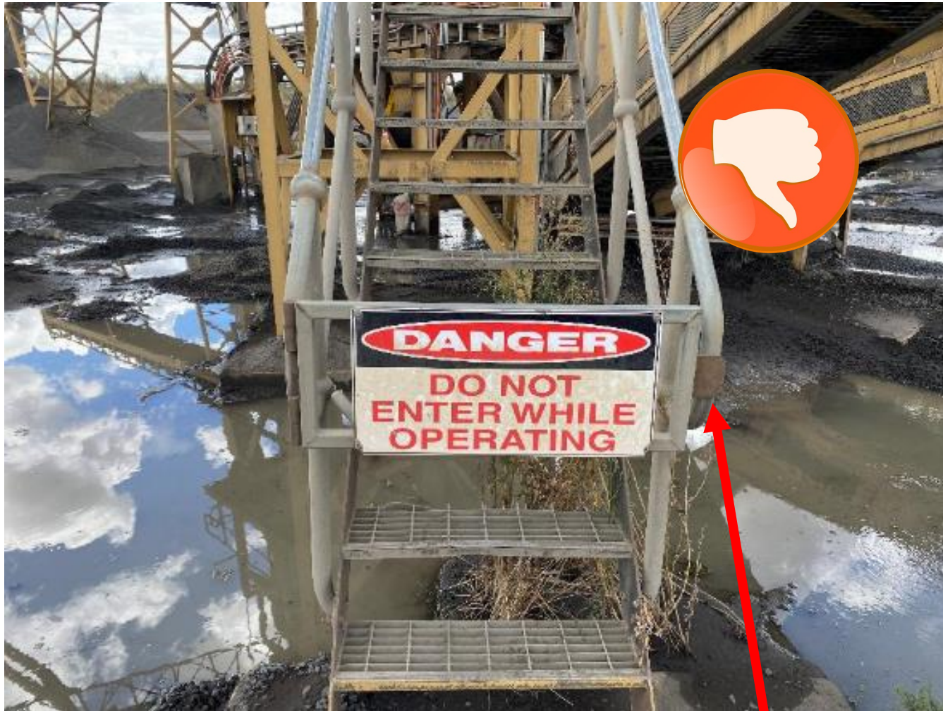
Barrier from entering an area – signposted but not secured
