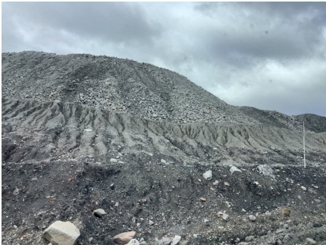
Figure 3 Rilling and erosion along high wall, south of Mini Strip TSF
