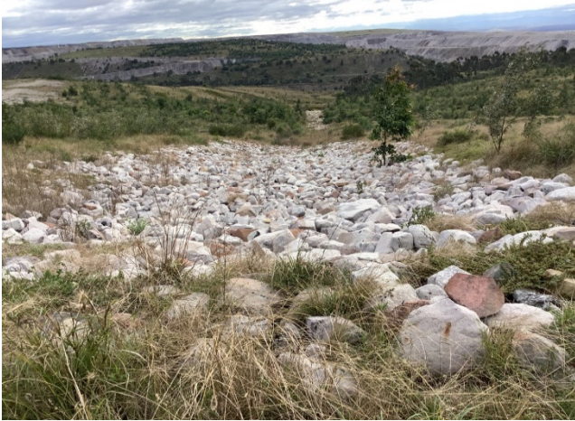
Figure 15 Green Mile drop structure
