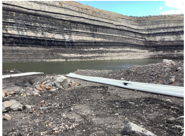
Figure 4 Overburden emplacement within Loders Pit TSF
