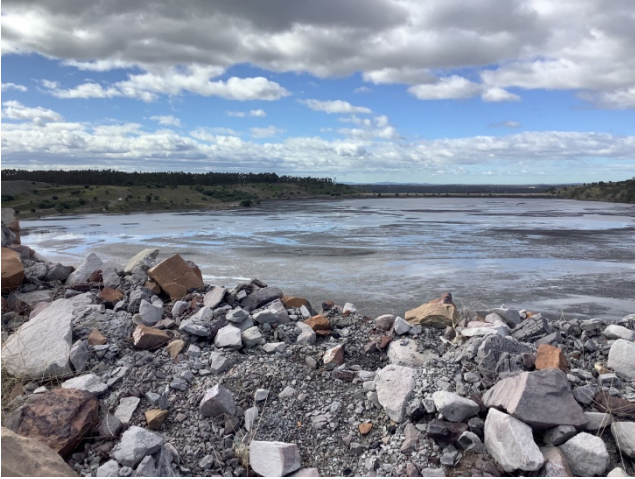
Figure 5 South Pit Centre Ramp tailings – Northern face
