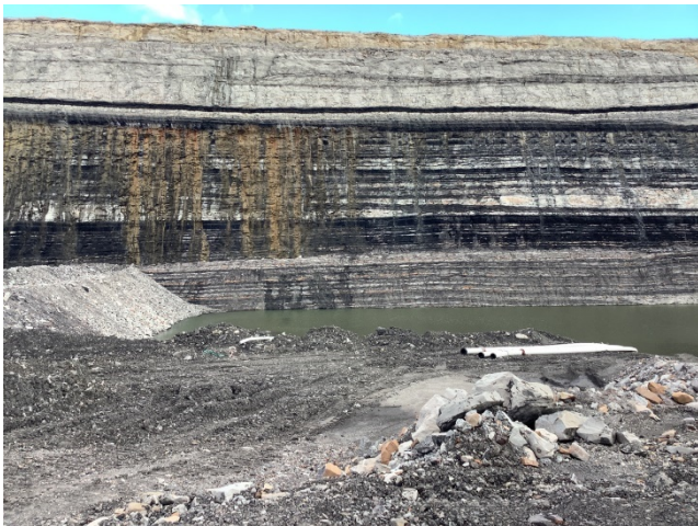
Figure 1 Potential AMD leachate within western wall of Loders TSF
