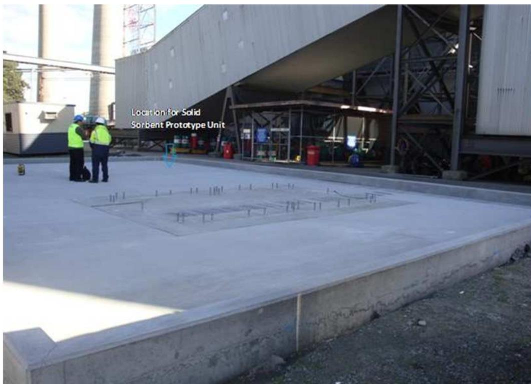
Figure 19: Concrete basement with proposed location for solid sorbent prototype test unit at power station
