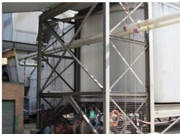
Figure 21: Photo of the constructed main flue gas supply and return lines from the flue duct
