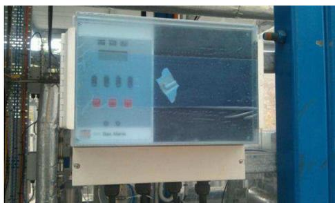
**Figure 28: Photo of the four channel hazardous gas detector installed on the solid sorbent test facility**
