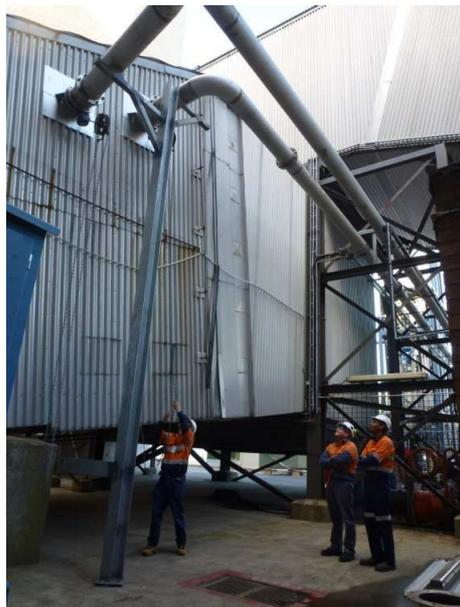
Figure 29: Opening of inlet flue gas pipeline on-site to provide flue gas to the solid sorbent test unit
