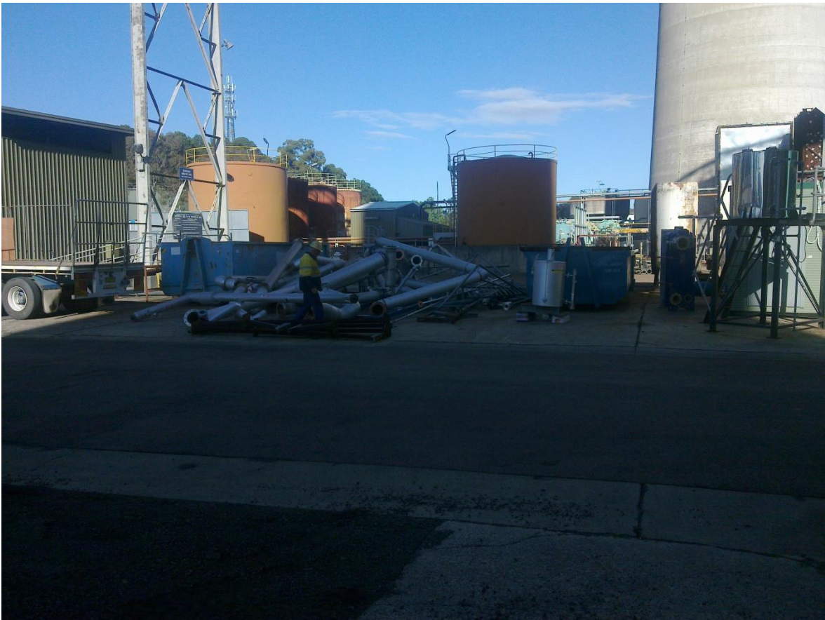
Figure 17 Pipework removed from the pilot plant
