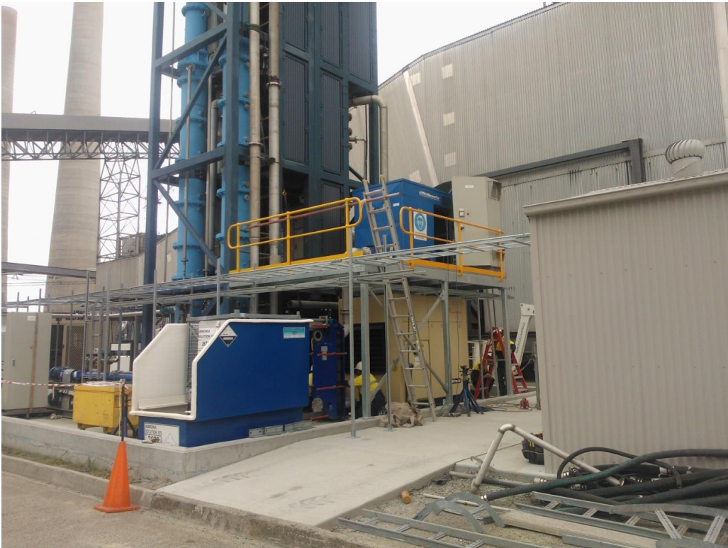
Figure 27 Chemical storage positioned
