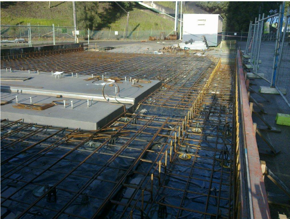
Figure 13 Forming up and setting reinforcement for main slab
