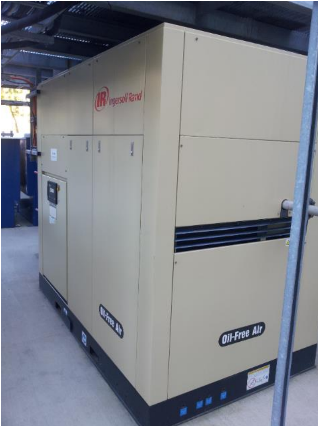
Figure 4 Compressor for pressurised absorption
