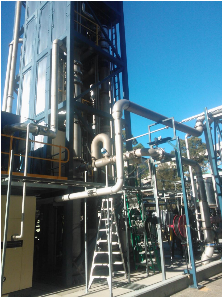
Figure 35 Installation of compressor and blower pipework and supports
