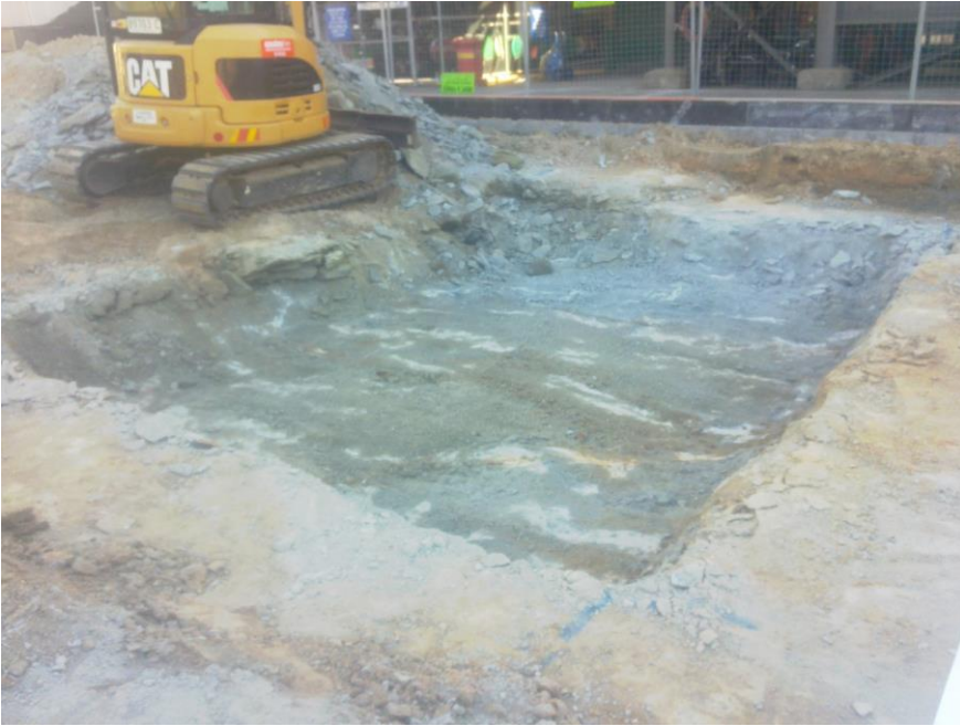
Figure 8 Excavation hampered by old concrete
