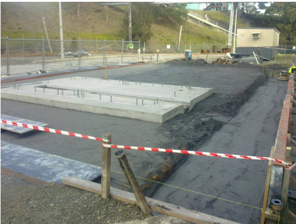
Figure 11 Preparation for main slab
