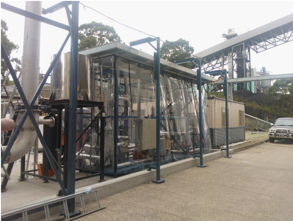
Figure 30 Pipework for connection of solid sorbent rig
