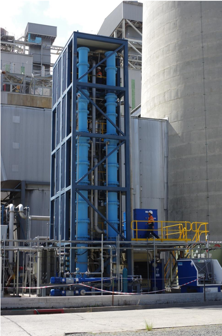
Figure 7 Absorbers with insulating ceramic paint
