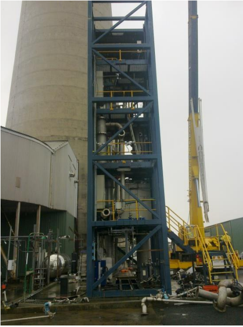
Figure 20 Dismantling of pilot plant
