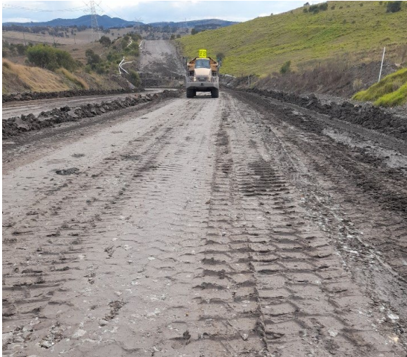
Figure 1 The Caterpillar 740 articulated truck involved in the incident
