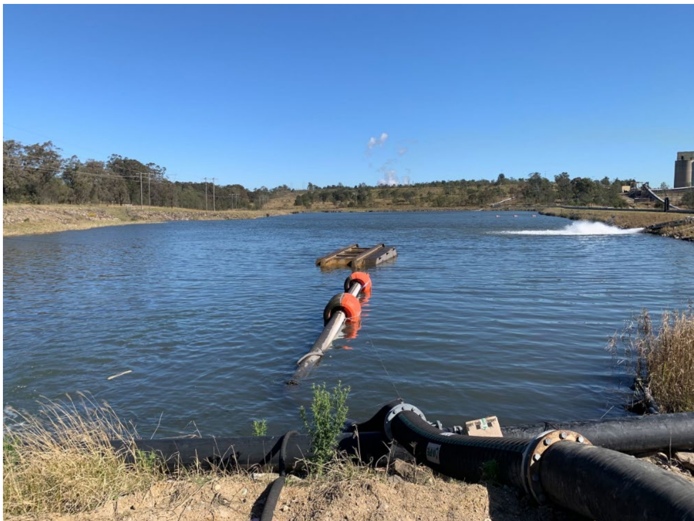
Figure 1 Pontoon on the dam after the incident
