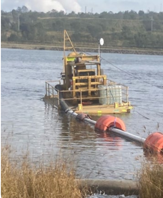
Figure 2 Pontoon on the dam before the incident
